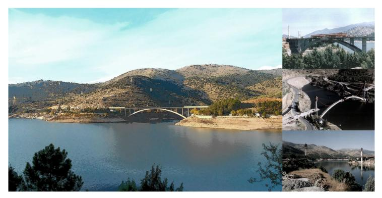
The Bridge over the El Burguillo Reservoir comprises a reinforced concrete arch 165.00m in span with a reinforced concrete upper deck 287.00m in total length. The solid arch is a constant 4.00m in width and has a variable depth running from 3.10 m at the abutments to 1.75 m at the crown. The deck comprises a solid slender 0.90 m deep section which consists of a 4.00m wide central core, coinciding with the width of the arch, and two large variable depth cantilevers each 4.00m in width.
